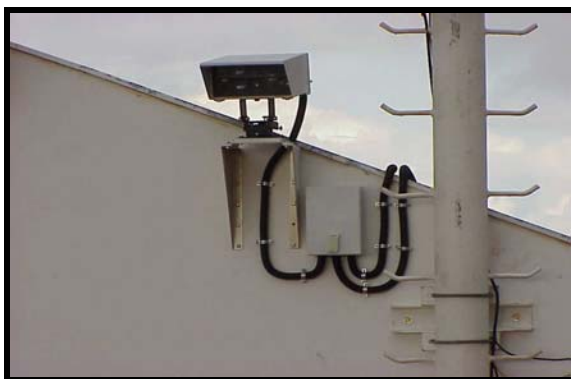
Figure 2.8: Wall Mounting (using JMP and JMB)
